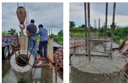
Fig. 4 Temporary beams fastening Dowel and test samples
