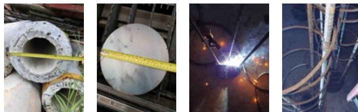
Fig. 3 The examination of the hollow hole size of PHC pile, Cutting Steel Plates, Dowel alignment and stirrup alignment
