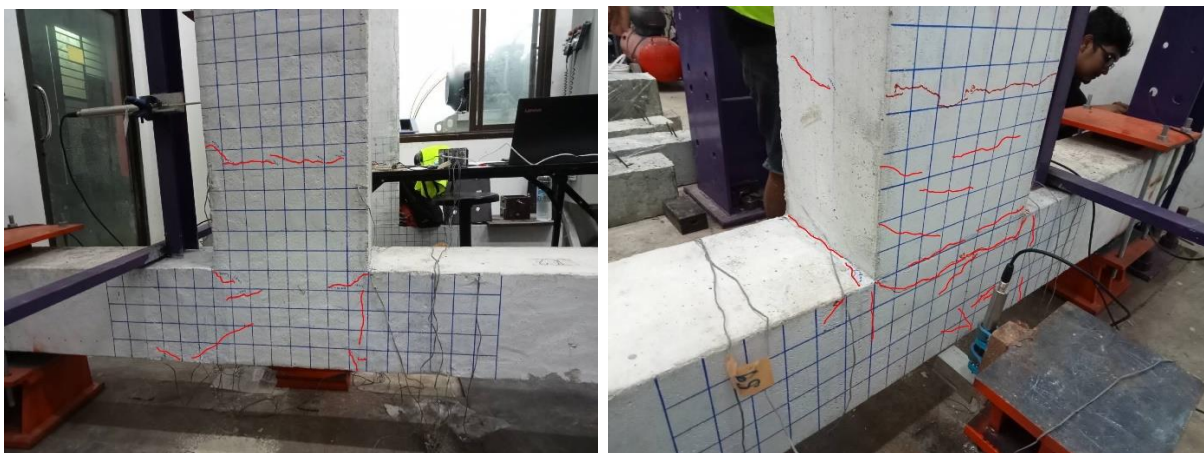
Fig. 7 Damage of the JC-1 and JC-1 PTMS specimen after testing.
