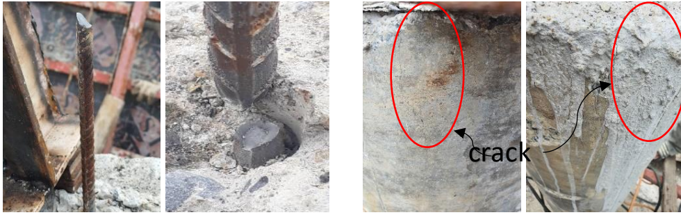
Fig. 7 (A) Failure of dowel bar in tensile force; (B) First cracks in concrete wall of the PHC piles
